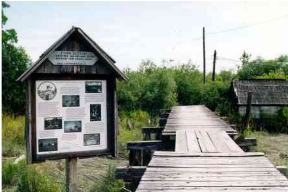
The only "draw bridge" in Richmond. When a new bridge was needed between Gilmour Island and the North bank of Finn Slough, the Anglo British Fishing Company donated all the required lumber. The fishermen gave their skills and labour voluntarily for the common cause. When a fisherman wants to take his boat through the "draw bridge" he simply draws four planks out, takes his boat through, and replaces the planks. The bridge was so well constructed in the 1940's that it is still in use today. Photo: Jouni Korkiasaari.
